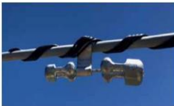
Figure 1: Stockbridge Damper
