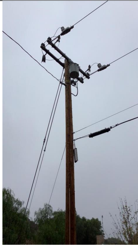
Item4GImg2: Overall view of the pole and covered conductor
