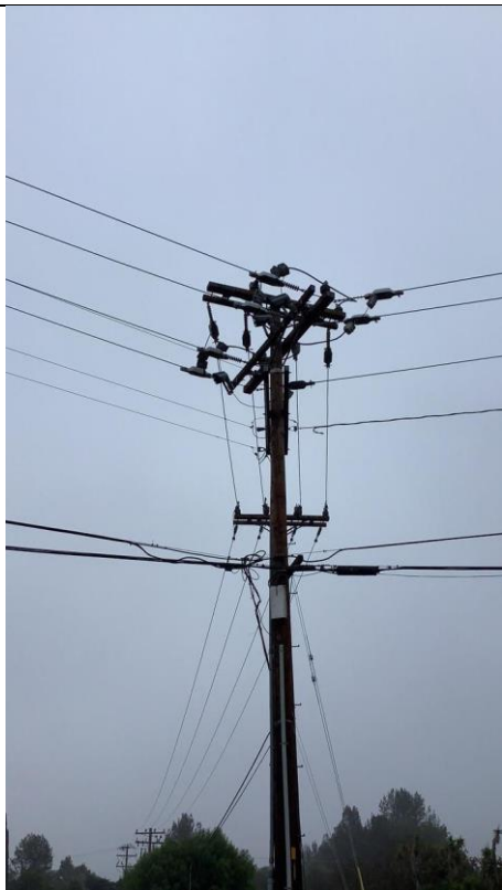
Item1G1mg2: Overall view of the pole and covered conductor
