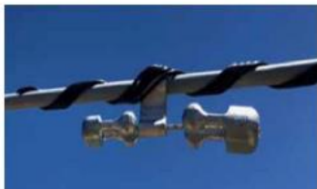
Figure 1: Stockbridge Damper
