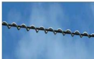
Figure 2: Spiral Damper
