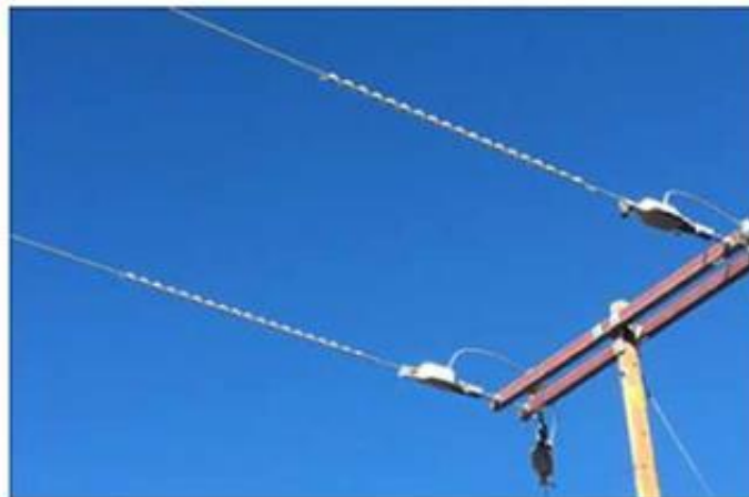
Figure CC 190-4: Installed Spiral Vibration Dampers on Covered Conductor
