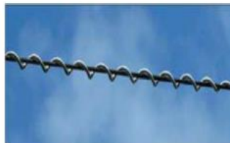
Figure 2: Spiral Damper
