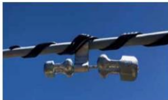
Figure 1: Stockbridge Damper
