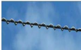
Figure 2: Spiral Damper
