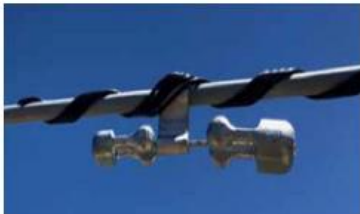
Figure 1: Stockbridge Damper
