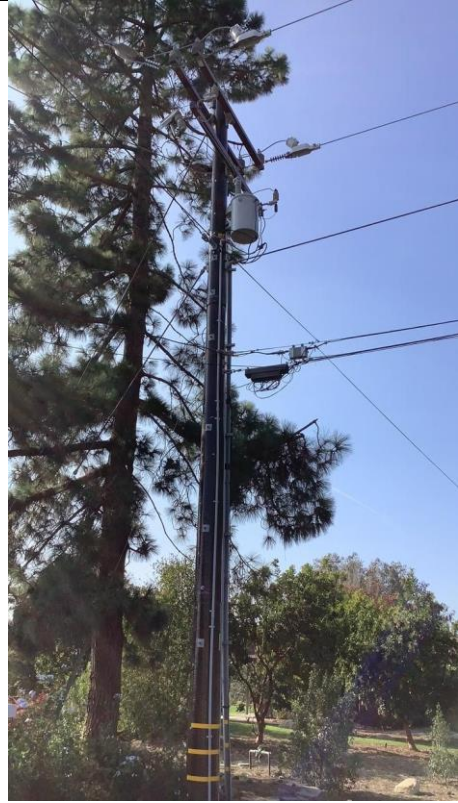
Item2Gimg2: Overall view of the pole and covered conductor installation.
