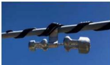
Figure 1: Stockbridge Damper
