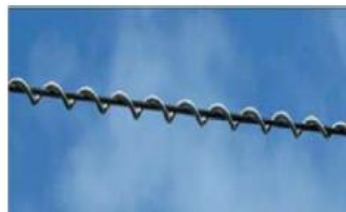
Figure 2: Spiral Damper
