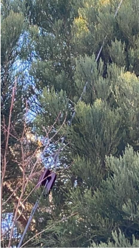
Item5GW2Img1: Vegetation touching guy wire above insulator
