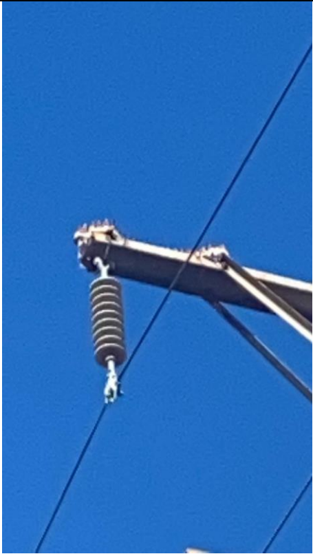
Item16IA1Img1: Bare conductor
