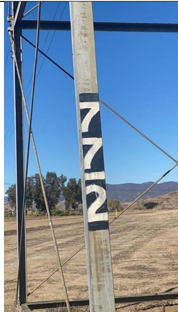
Item16IA2Img2: Other structure ID
