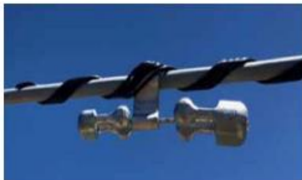
Figure 1: Stockbridge Damper
