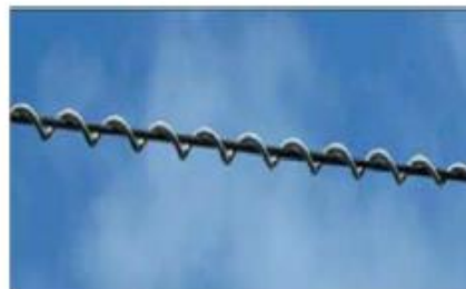
Figure 2: Spiral Damper
