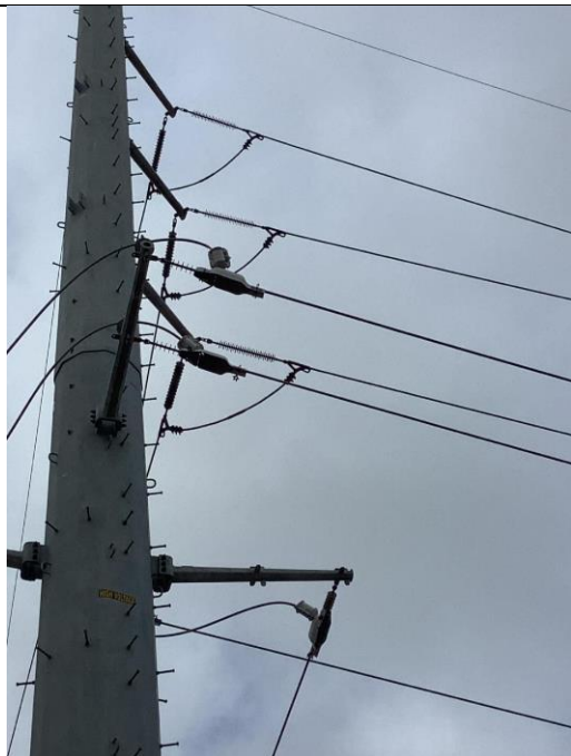
Item20IA1img1: No vibration dampers installed
