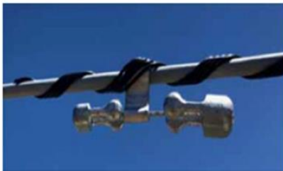
Figure 1: Stockbridge Damper
