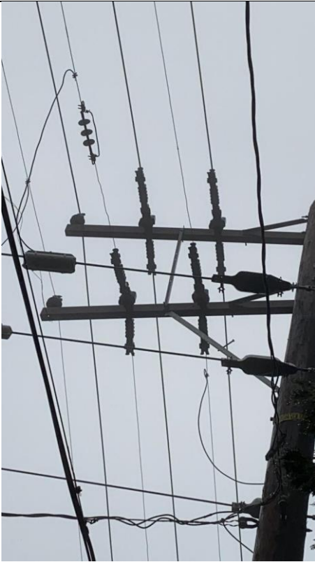
Item1IA1Img1: Top level crossing phase showing bare wire and no covered conductor installed
