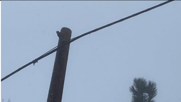
Item9IA1img1: Close up no covered conductor
