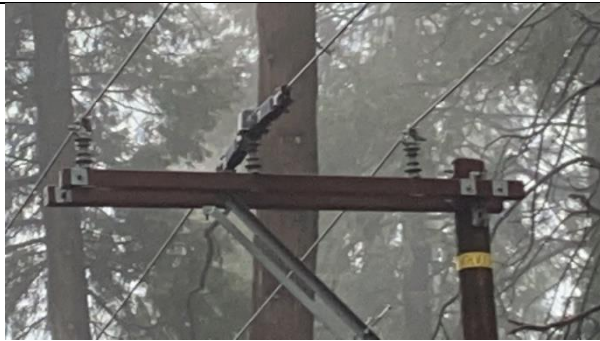
Item6IA2Img1: Overall view of insulators with cover. Insulators should be vice top polymer pin type insulators with nylon inserts
