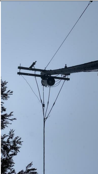
Item11IA1img1: No covered conductor installed
