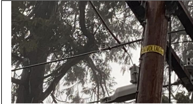
Item3IA4Img1: Bare dead-end conductor with no cover
