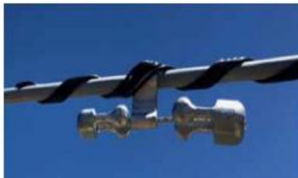
Figure 1: Stockbridge Damper
