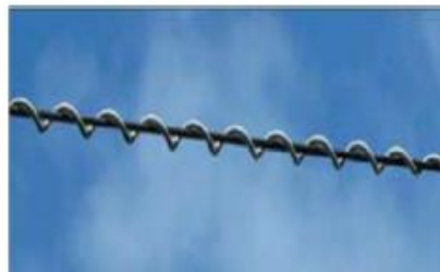
Figure 2: Spiral Damper
