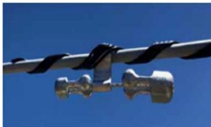
Figure 1: Stockbridge Damper
