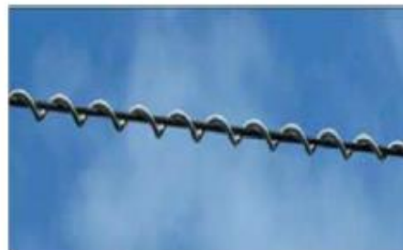
Figure 2: Spiral Damper
