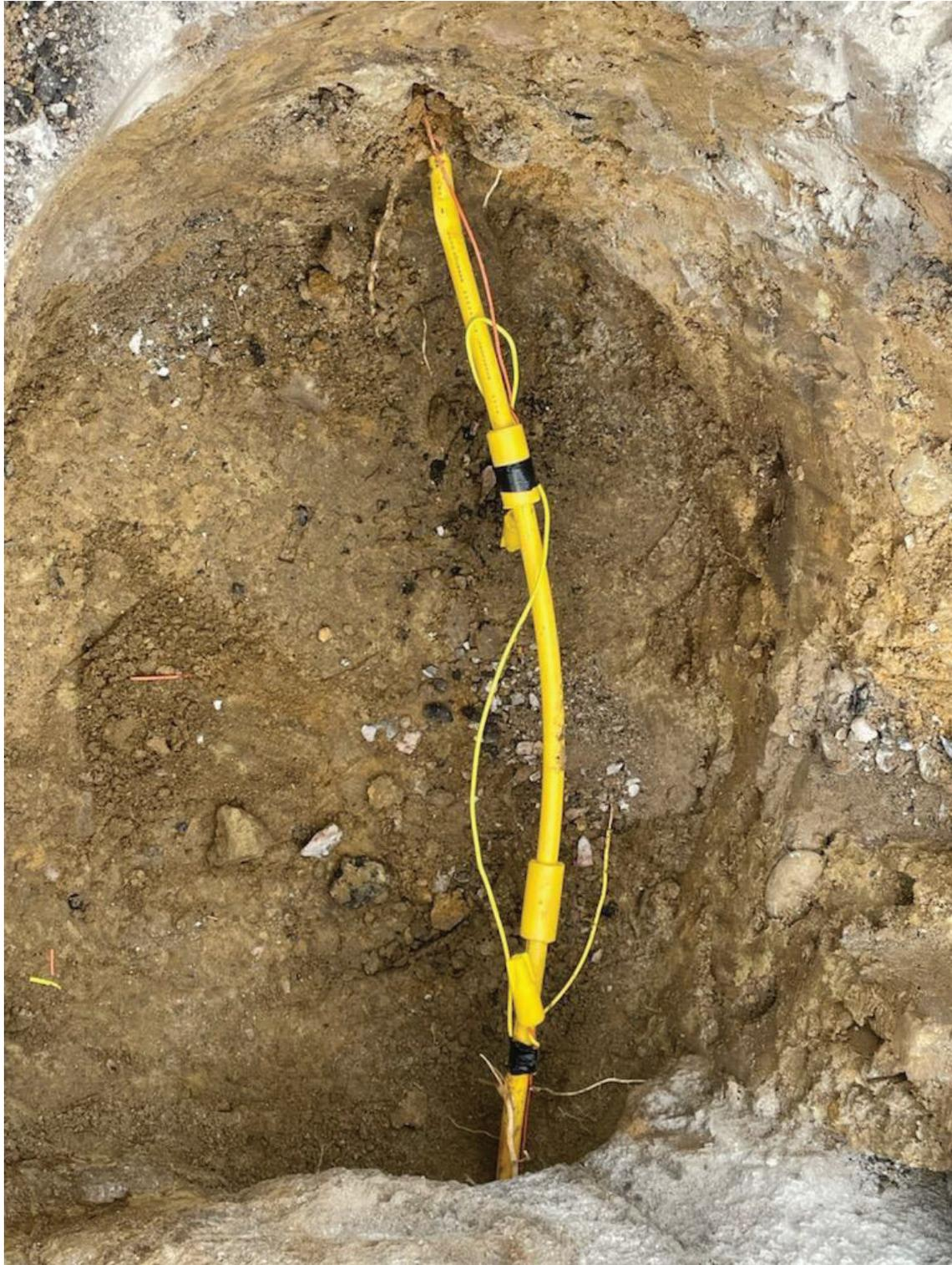
Photo 4 (Courtesy SDG&E) Line and Tracer Wire Repair
