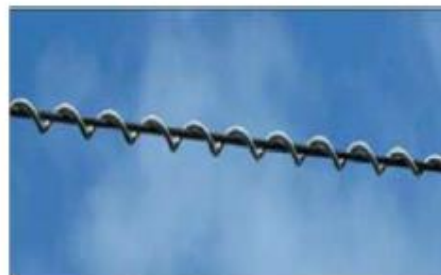
Figure 2: Spiral Damper
