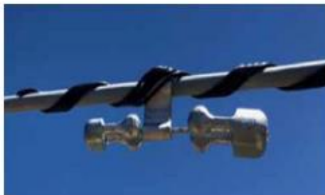
Figure 1: Stockbridge Damper
