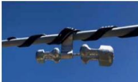
Figure 1: Stockbridge Damper
