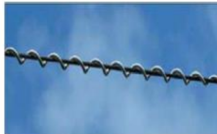
Figure 2: Spiral Damper
