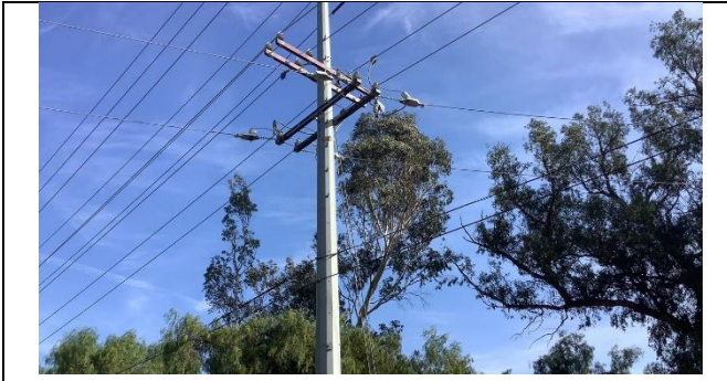
Item9IA2Img1: Overall pole
