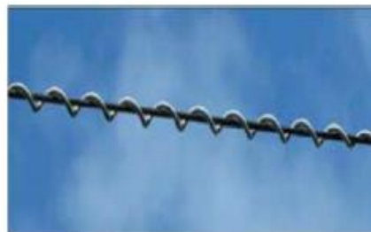
Figure 2: Spiral Damper
