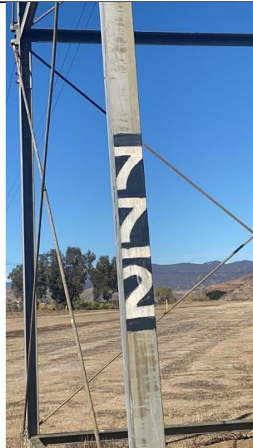
Item16IA2Img2: Other structure ID
