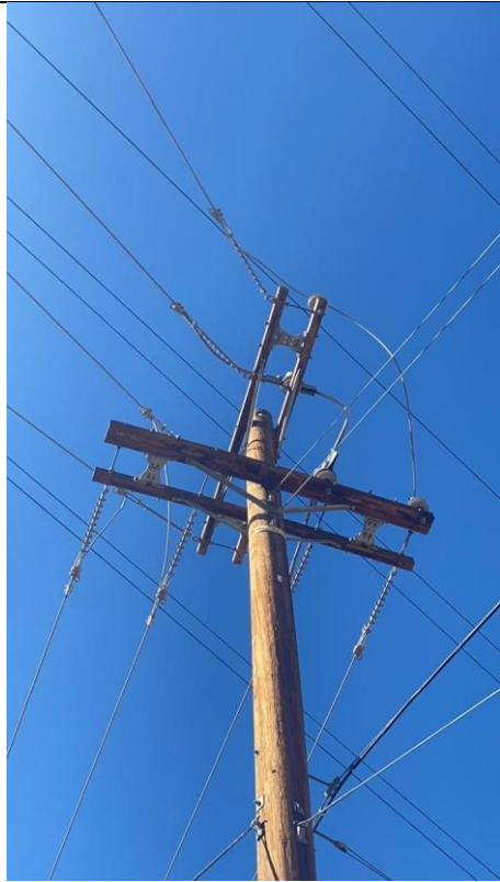
Item15IA1img2: Overall pole
