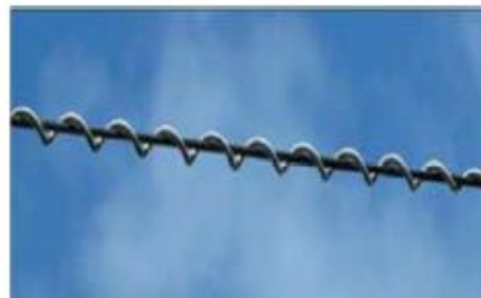
Figure 2: Spiral Damper
