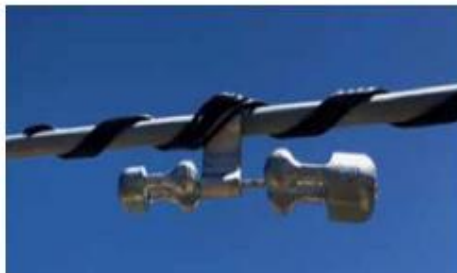
Figure 1: Stockbridge Damper
