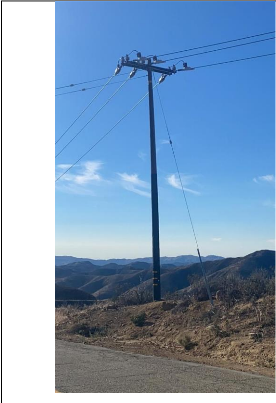
Item11GImg1: Overall pole
