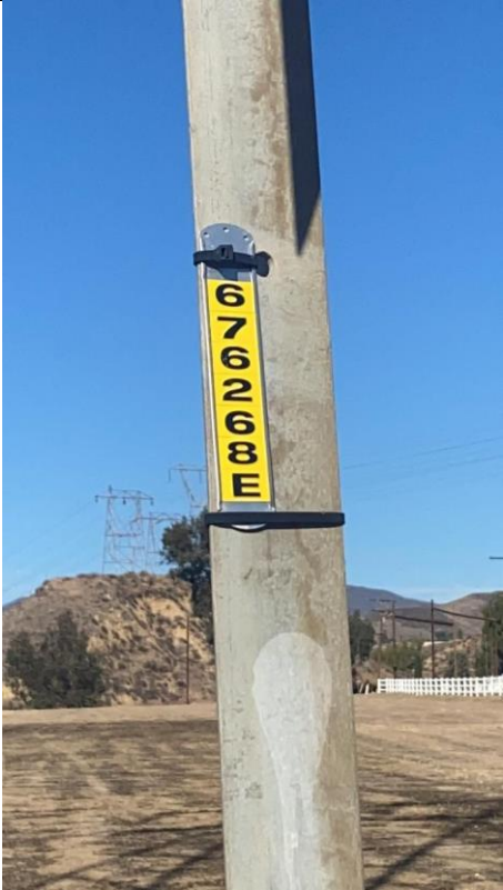
Item16GImg2: Structure ID
