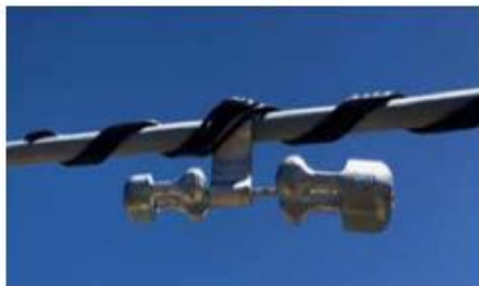
Figure 1: Stockbridge Damper
