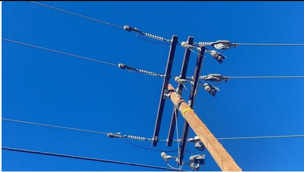
Item2IA3Img1: No bolted wedge connector covers when transitioning from bare to covered conductor
