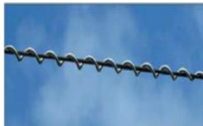
Figure 2: Spiral Damper
