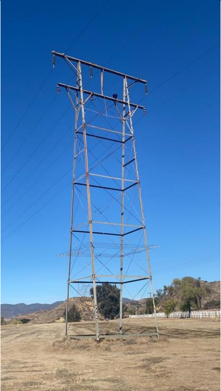
Item16GImg1: Overall structure
