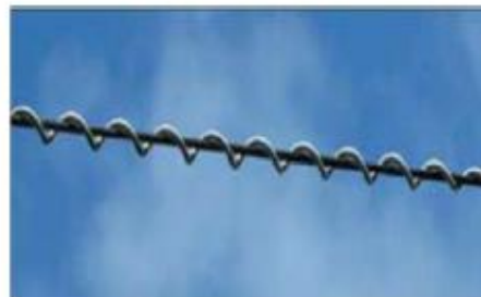
Figure 2: Spiral Damper
