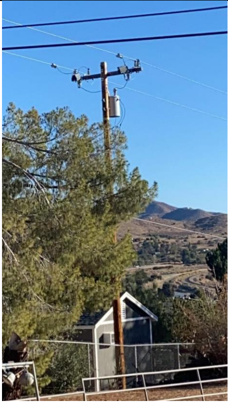
Item5GIimg1: Overall pole
