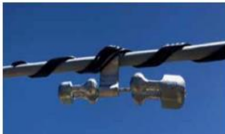
Figure 1: Stockbridge Damper
