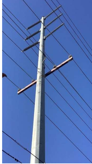
Item1GImg2: Overall view of the pole and covered conductor
