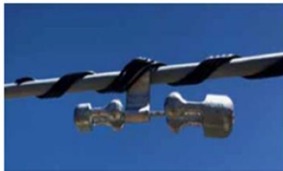
Figure 1: Stockbridge Damper
