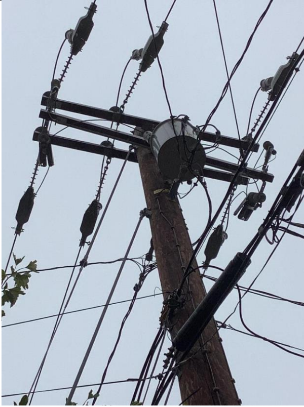
Item1IA1mg1: Vibration dampers are missing
