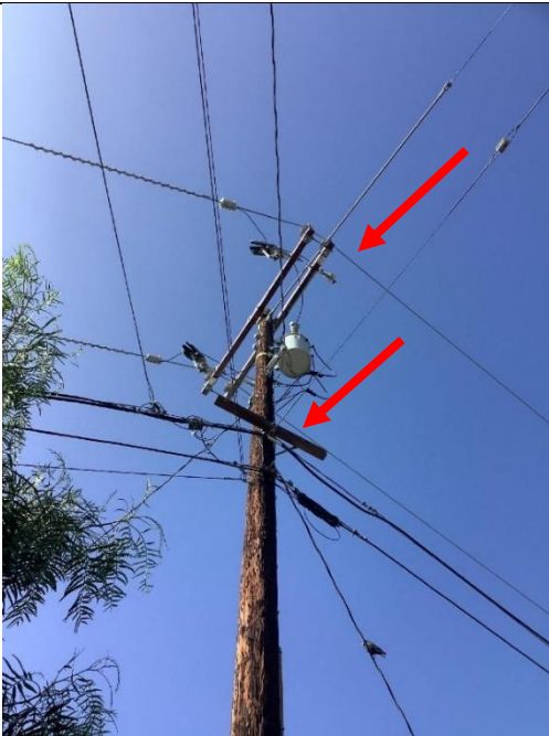
Item8IA1mg1: One side vibration dampers installed
