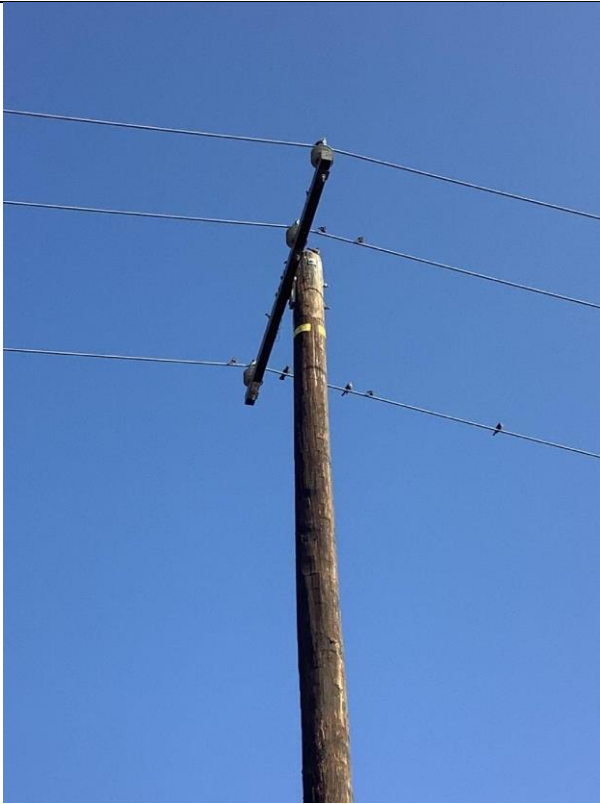
Item10IA1mg1: Vibration dampers are missing
