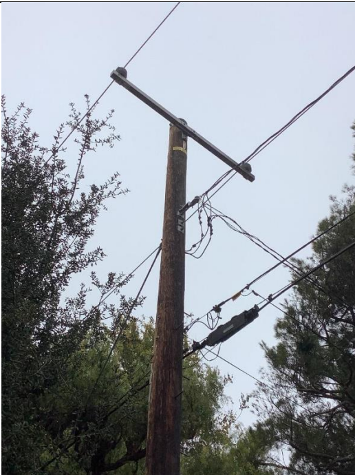
Item6IA1mg1: Vibration dampers are missing
