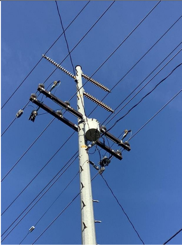
Item12IA1mg1: Vibration dampers are missing
