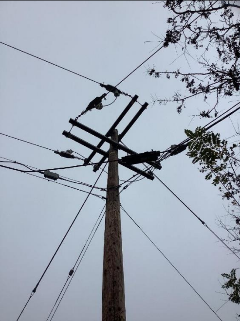
Item4IA1Img1: Vibration dampers are missing
