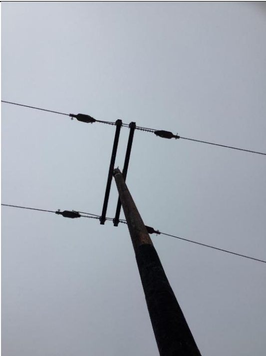
Item7IA1mg1: Vibration dampers are missing
