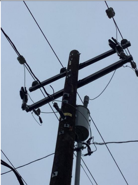
Item2IA1Img1: Vibration dampers are missing
