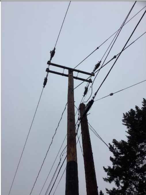
Item5IA1Img1: Vibration dampers are missing
