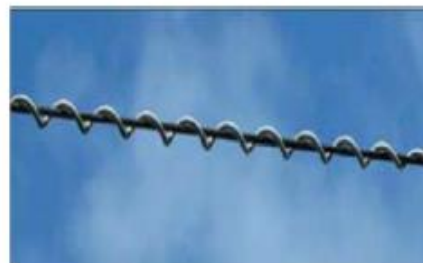
Figure 2: Spiral Damper
