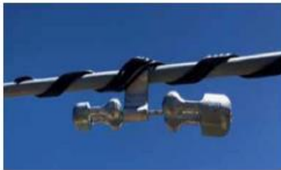
Figure 1: Stockbridge Damper
