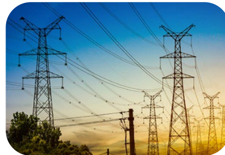
Detailed overhead visual inspections
