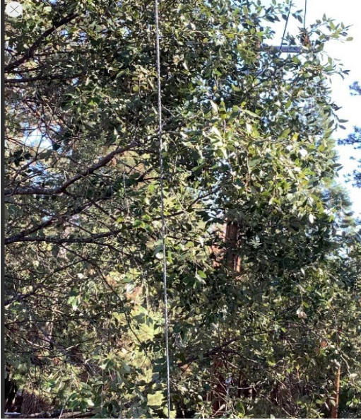
Photo 1: Picture of vegetation contacting the guy wire
