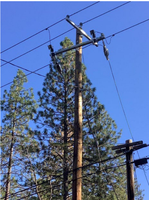
Photo 2: Picture of the entire pole
