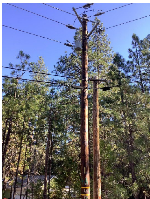
Photo 2: Picture of the entire pole
