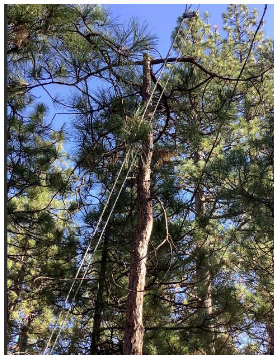
Photo 3: Picture of vegetation contacting the guy wire
