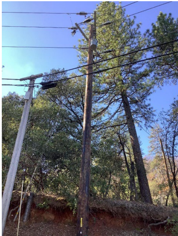
Photo 2: Picture of the entire pole
