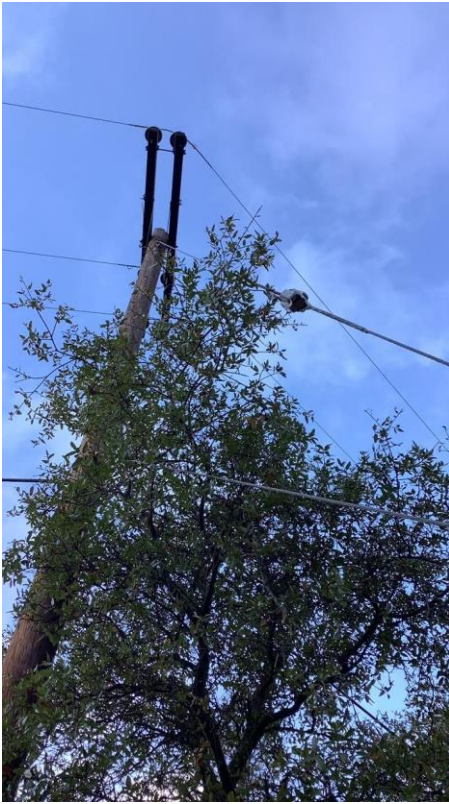
Figure 4 Item13GW2Img2: Photo of Interior Live Oak branches touching guy wire above insulator
