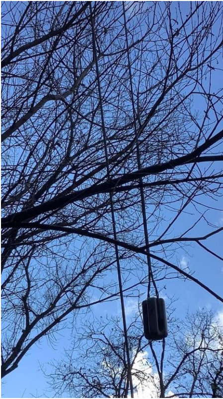
Figure 2 Item9GW2Img2: Photo of branches intertwined with guy wire above insulator
