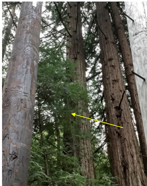
Photo 3: Picture of vegetation contacting the guy wire
