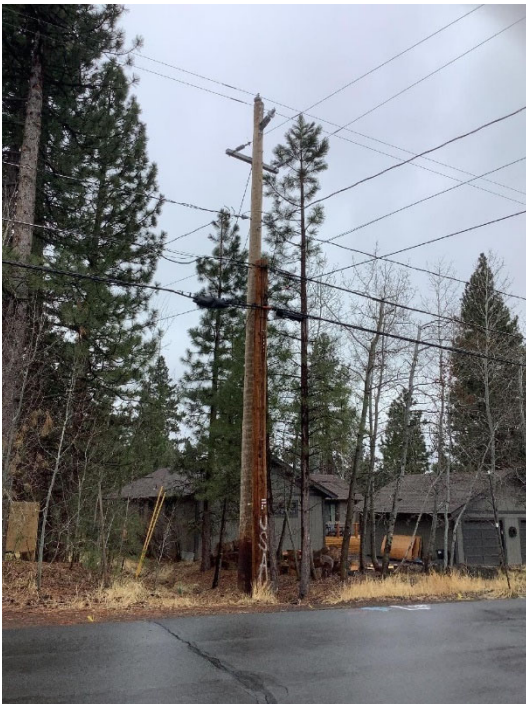
Item5CD6Img3: Overall utility pole
