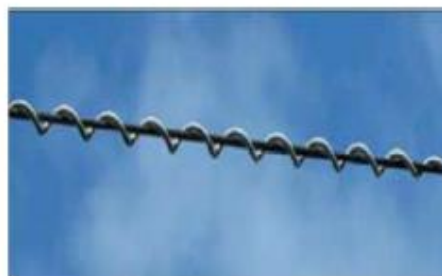
Figure 2: Spiral Damper
