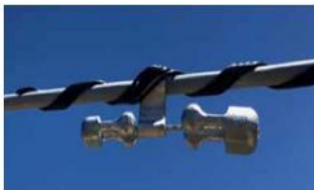
Figure 1: Stockbridge Damper
