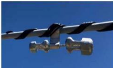
Figure 1: Stockbridge Damper
