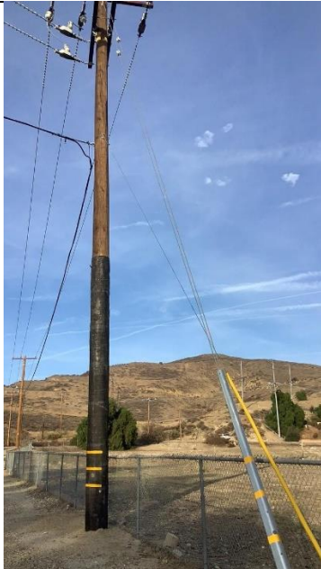
Item11IA1Img1: Overall view of down guy
