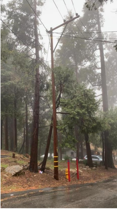
Item2GImg1: Overall pole
