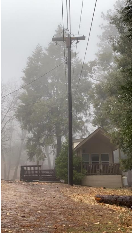
Item11GImg1: Overall pole
