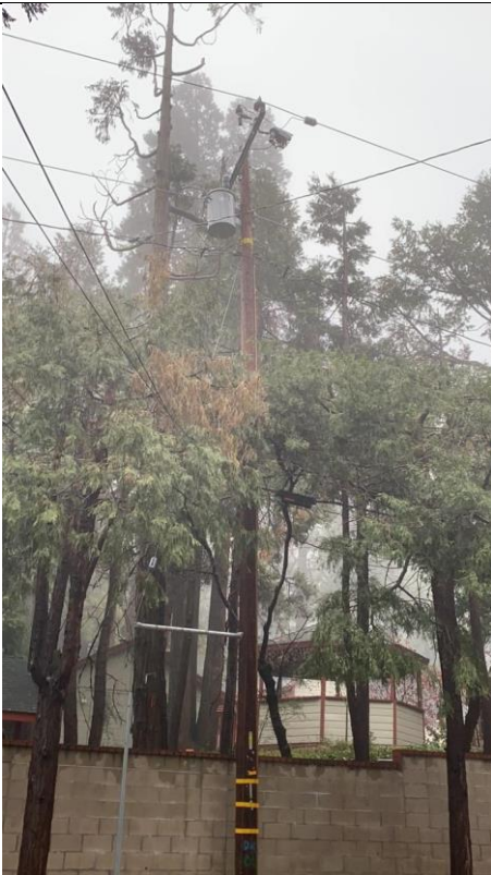
Item7G1mg1: Overall pole
