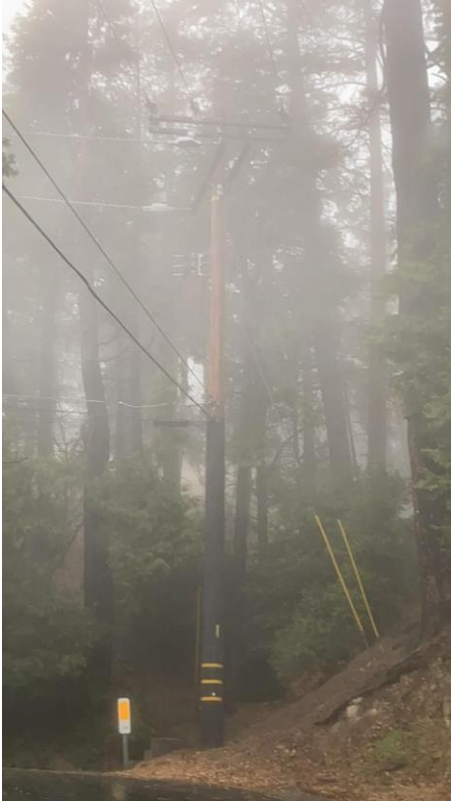
Item8GImg1: Overall pole
