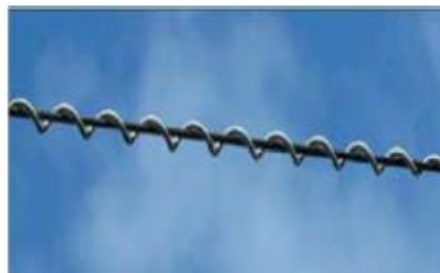
Figure 2: Spiral Damper
