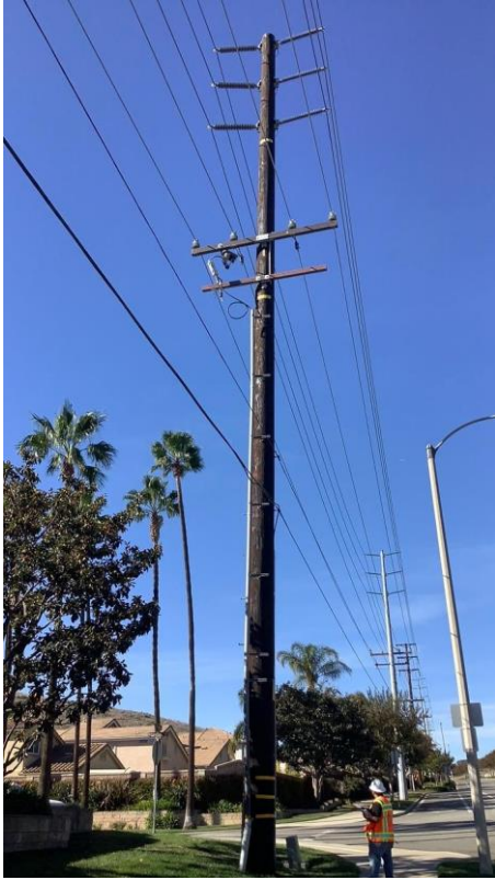
Item5GImg1: Overall view of pole
