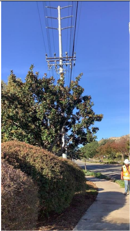
Item1IA2Img1: Overall pole
