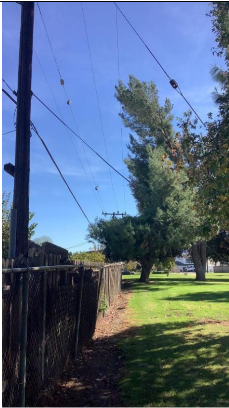
Item7CD4Img1: Overall view of pole looking East containing three splices
