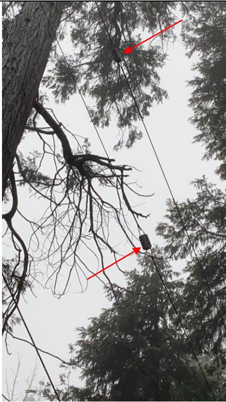
Item4IA2Img1: Porcelain insulator on down guy wire
