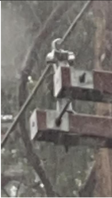
Item5IA3Img1: Close up view of insulator. Should be vice top polymer pin type insulators.
