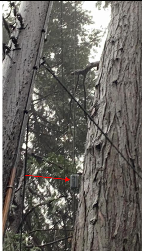
Item4IA2Img2: Third porcelain type down guy insulator
