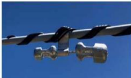
Figure 1: Stockbridge Damper
