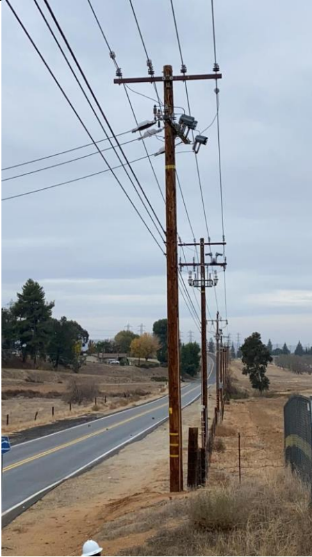
Item12GImg1: Overall pole
