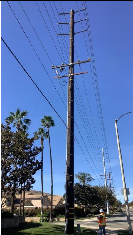
Item5GImg1: Overall view of pole
