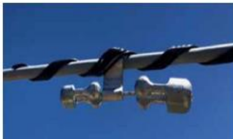
Figure 1: Stockbridge Damper
