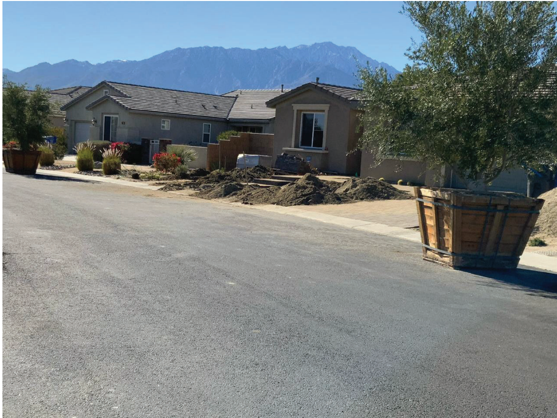
Photo 1 – Area of Excavation (photo provided by SoCal Gas)
