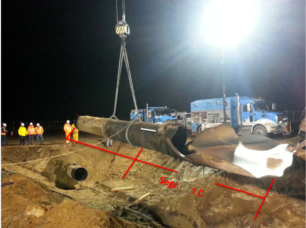
Figure 10. A photograph of Segment C and Segment D.
