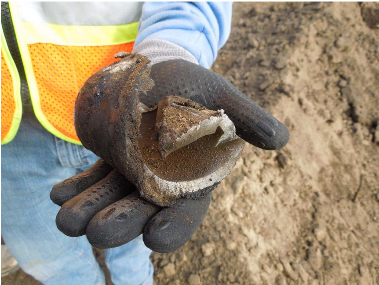
Figure 3. A photograph of a metal section resulting from the ripper attachment striking the pipeline.
