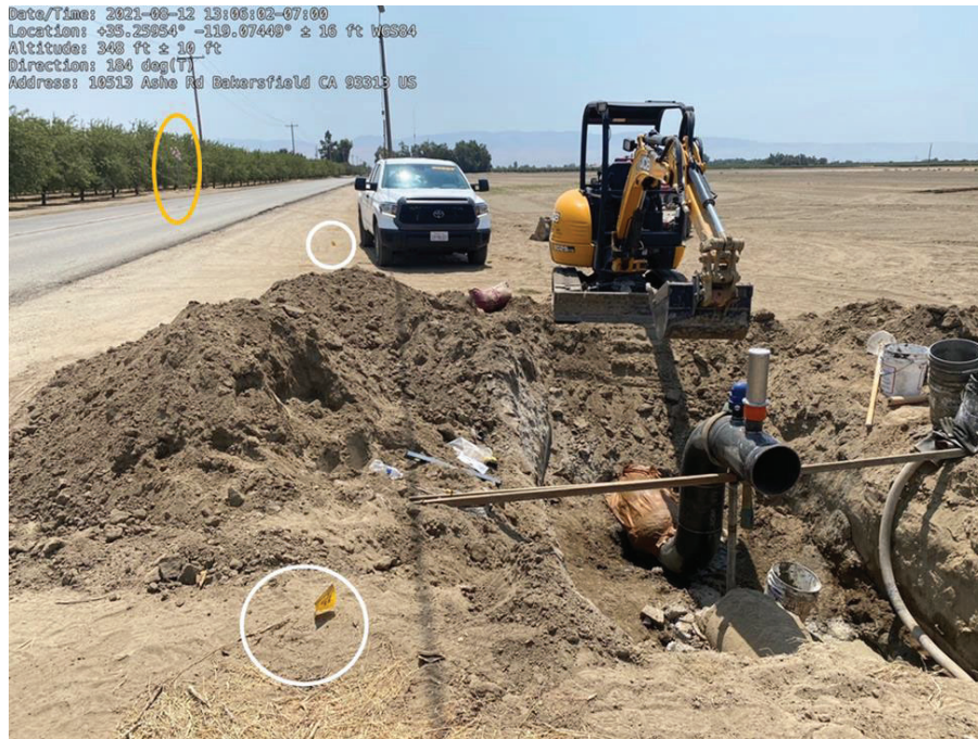
Figure 2: From Exhibit 1 , image of excavation area. In the foreground, to the bottom right, can be seen an old gas/petroleum temporary marking flag (circled in white). More difficult to see, to the left of the white truck, is (possibly) another yellow gas/petroleum marking flag (circled in white). In the top left of the photo, just to the left of the utility pole on the opposite side of the street, is a partially obscured diagonal permanent pipeline marker representing the location of a PG&E transmission pipe (orange oval). Photograph provided by Crimson Pipeline. White circles and orange oval added for clarity.
