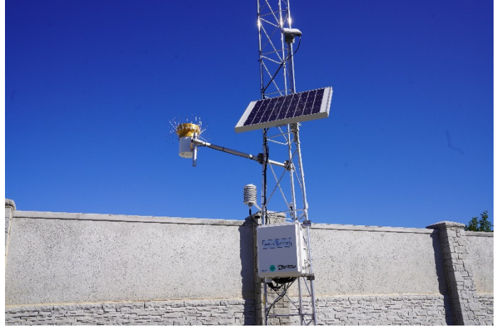
269 Weather Station, Exterior, View North, Close up
