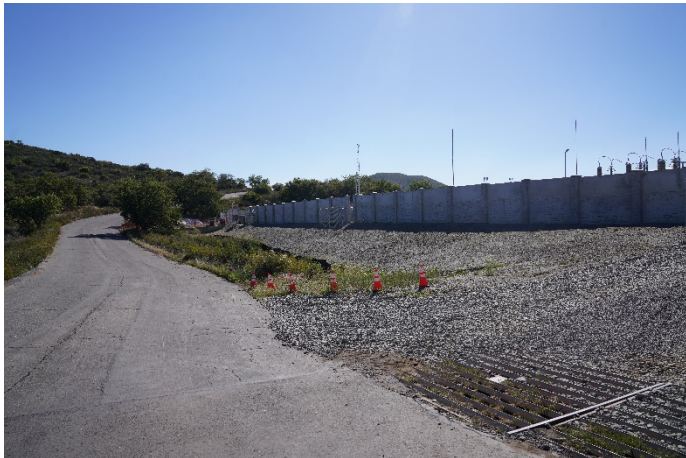
302 West Wall, Exterior, View East
