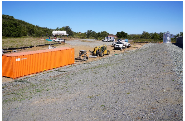
314 West Wall, Exterior, View Northwest
