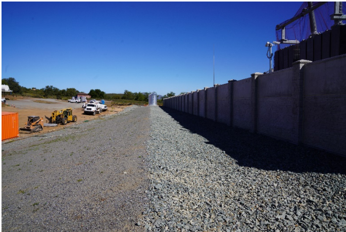
312 West Wall, Exterior, View North
