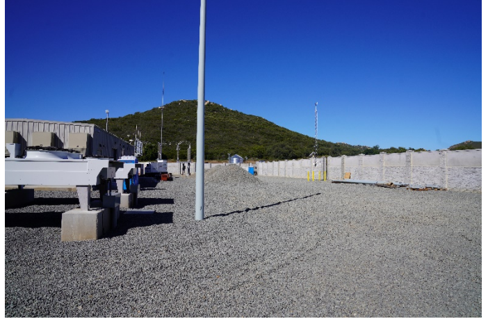
293 North Wall, Control House, View Southwest
