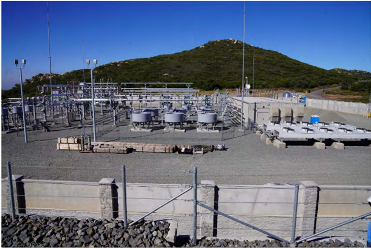
Figure 9. North Exterior Wall and Yard
