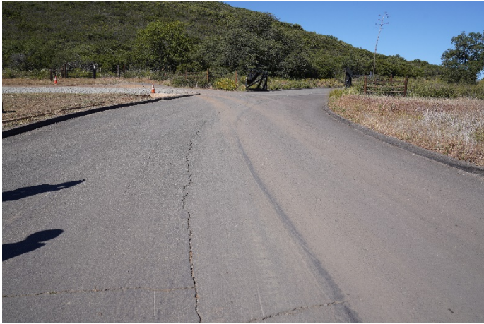
307 Access road, View Northwest
