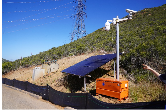
317 Overhead Transmission Line (OHTL) beyond foundation
