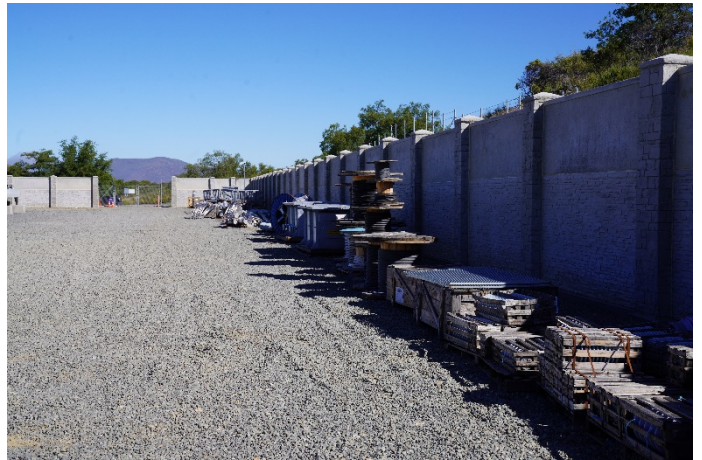
287 Interior East wall, View North
