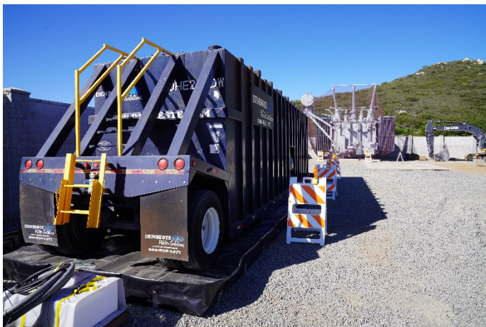
278 Denbeste Water Solutions trailer, View Southwest
