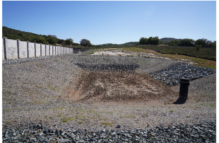
311 West Wall, Exterior, Catch basin, Wide angle View SE
