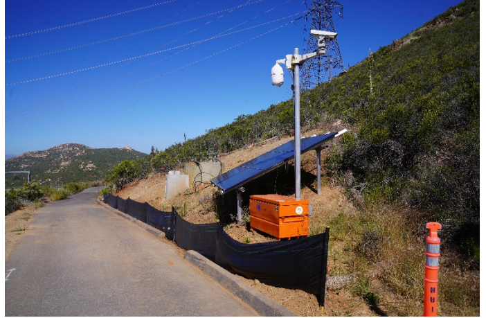
330 OHTL beyond foundation for single pole, View West
