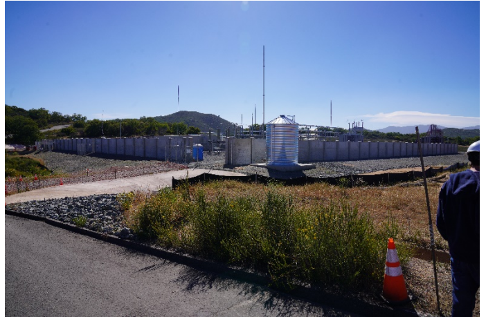
308 Fire Dept. Water Tank, NE corner, Exterior, Wide View SE
