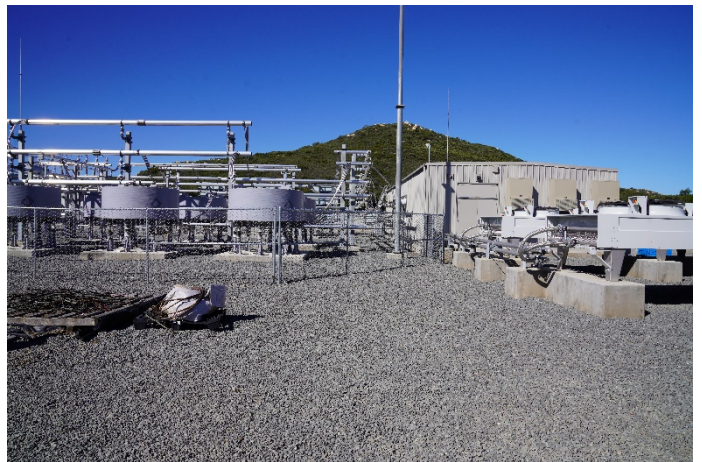
289 Reactors, Control House, View Southwest
