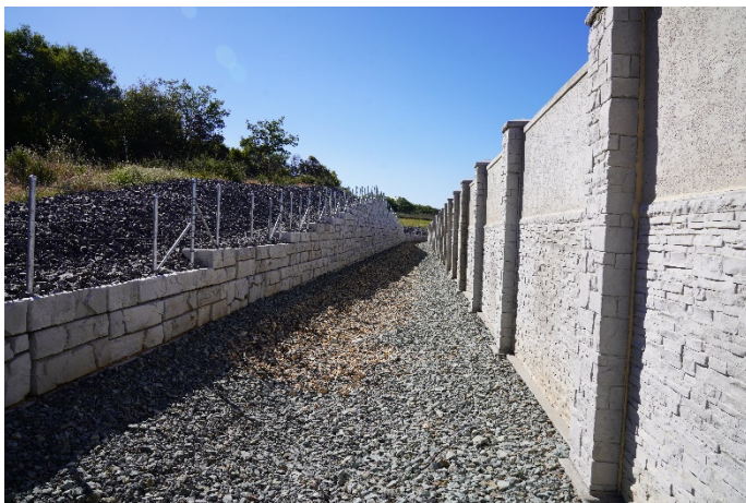
296 East Wall, Exterior, View South
