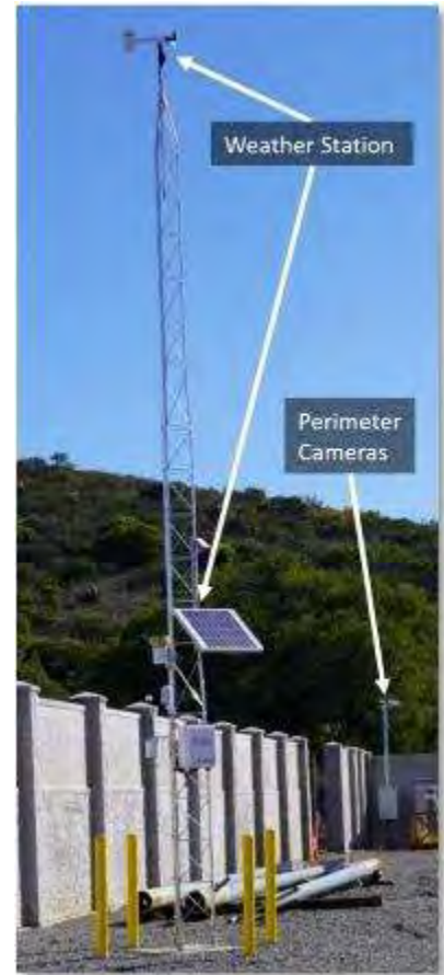
Figure 2. North Wall, Weather Station
