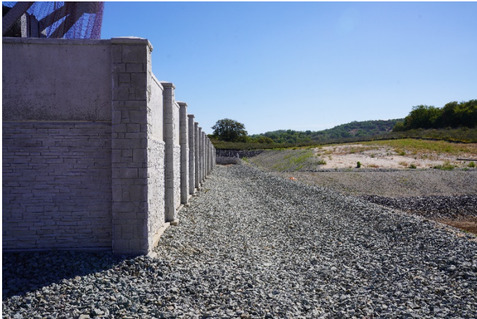
309 West Wall, Exterior, View Southeast
