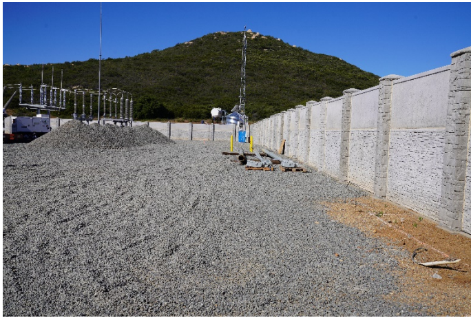
294 500-kV Cable risers, Interior North Wall, View West
