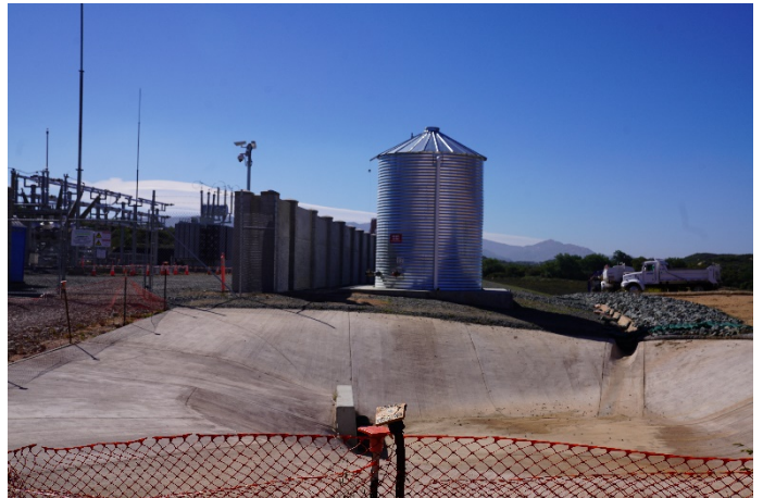
303 Fire Department Water Tank, West, Exterior, View South
