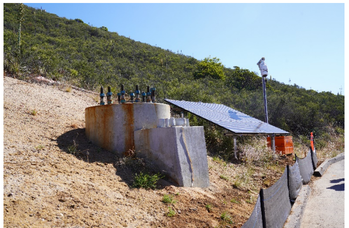
325 Foundation for single steel pole, security camera
