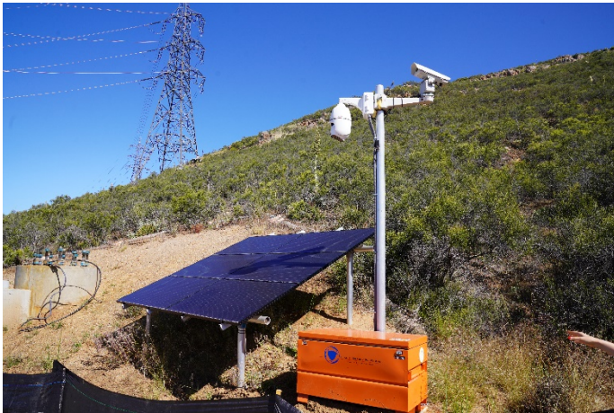
318 OHTL beyond foundation, security camera, View West
