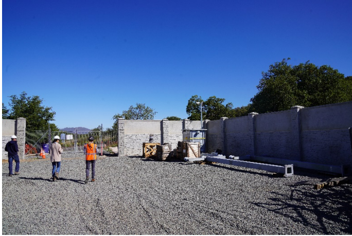
292 North Wall, Interior, Gate, View North
