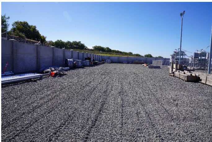
290 East Wall, Interior, View South
