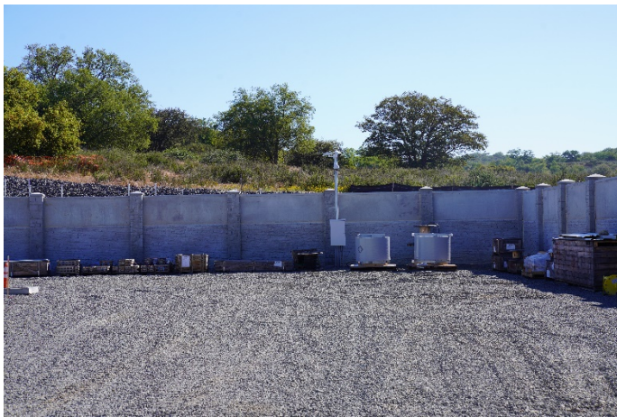
276 Cameras, reactors, View South, close up
