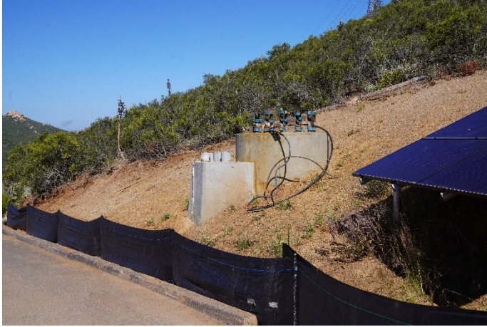
316 Foundation for single steel pole
