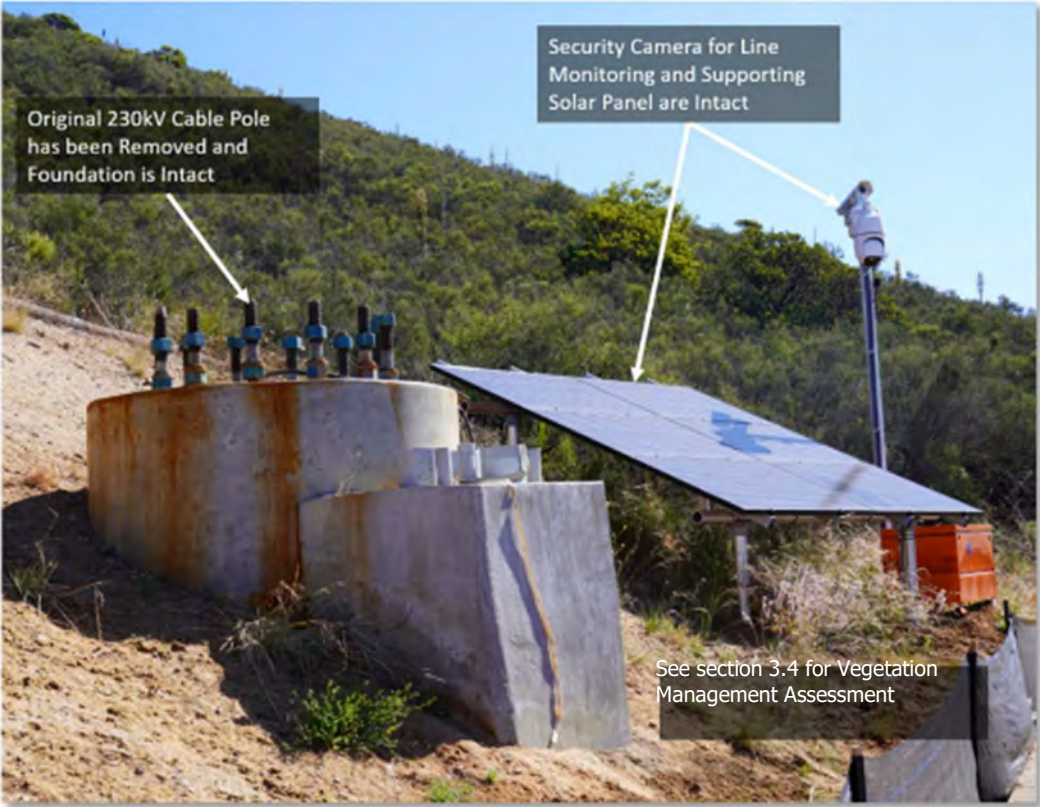
Figure 7. Foundation for Single Steel Pole, Security Camera
