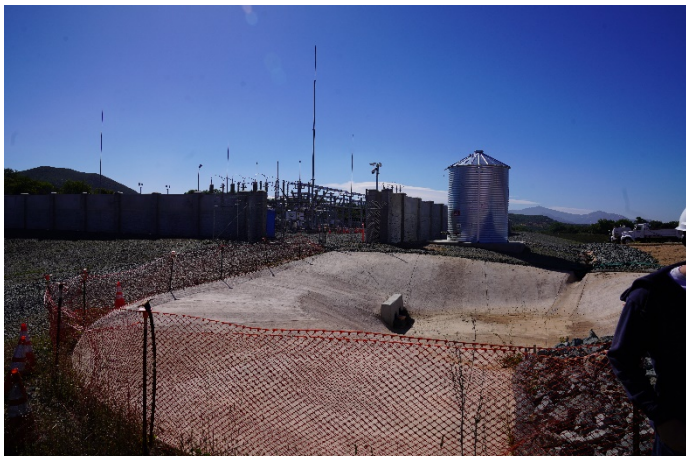
304 Fire Dept. Water Tank, NW corner, Exterior, View SE
