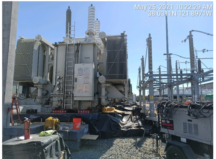
4 Transformer Seismic Upgrades
