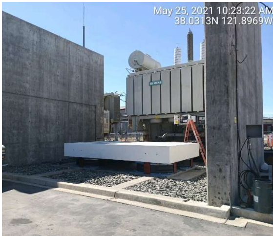
Figure 6. Seismic Retrofit for Transformers.
