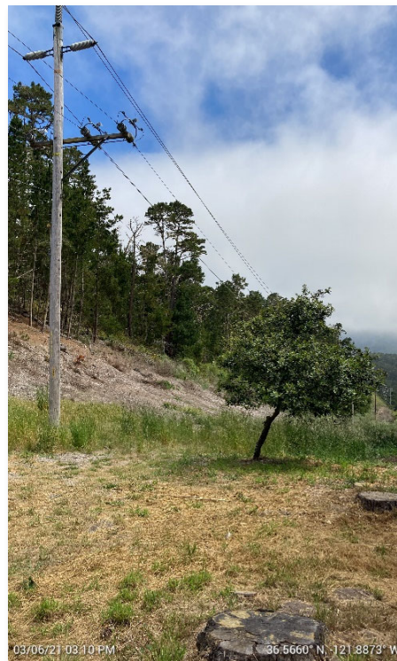
Figure 29: Site work included tree and slash removal.
