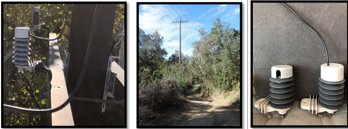
Figure 7 (a) Concealed lightning arrester (b) ductile iron pole (c) comparison of lightning arrester models
