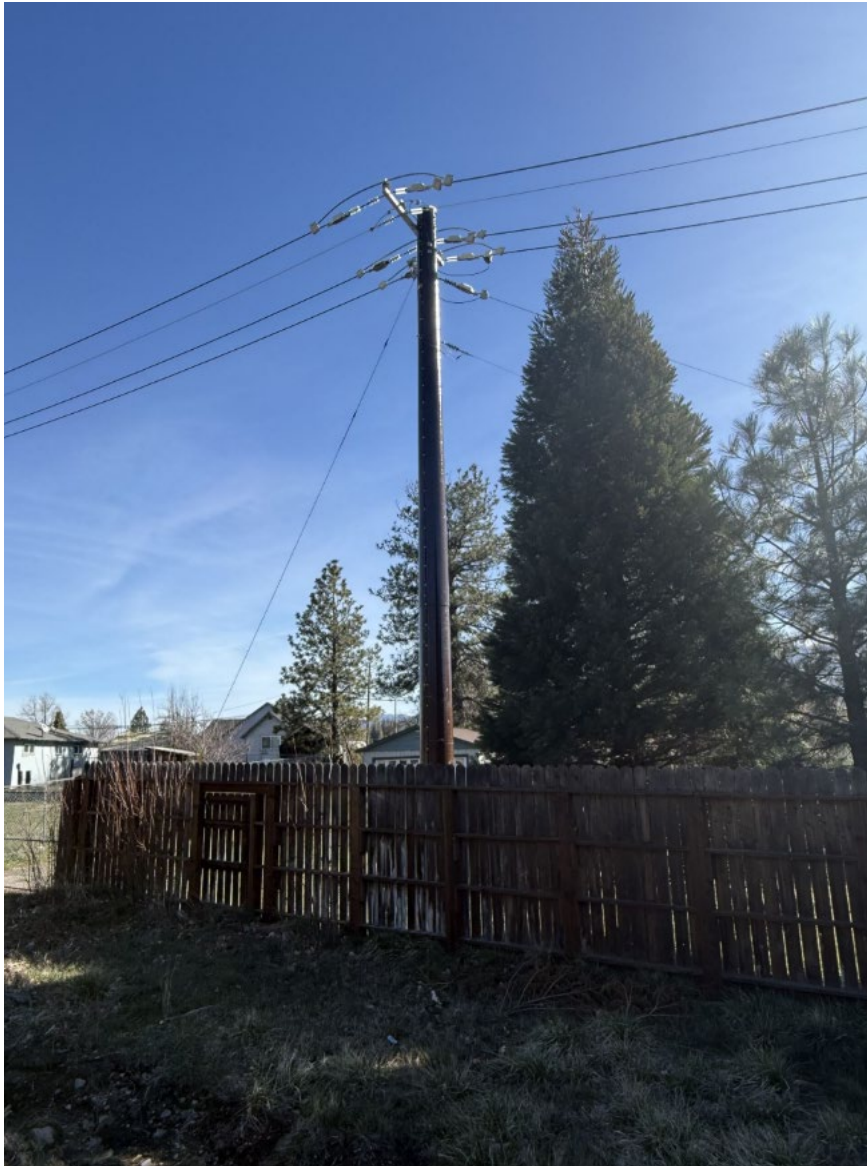
Picture 1: Near Grid Hardening ID 8077661 at coordinates 41.4293338392048, -122.389120, Picture taken March 12, 2026.
