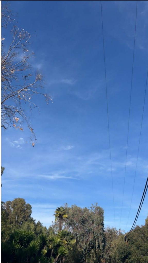
Photo 3: Photo showing the proximity of the dying eucalyptus tree branches (left) to the conductors (right).
