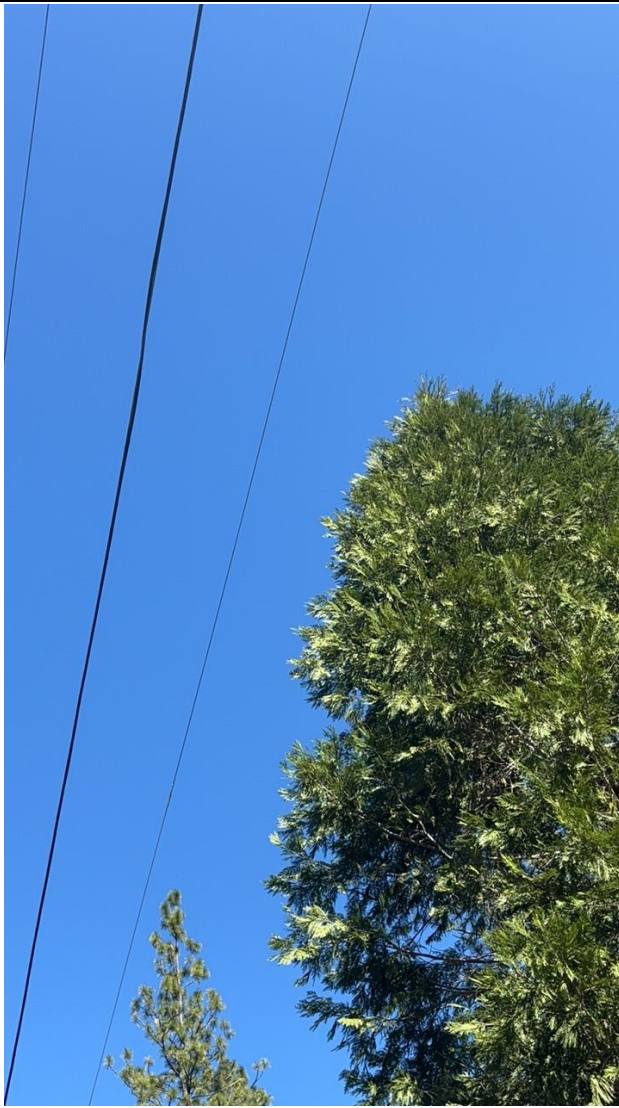
Photo 3: Close-up photo of the same cedar tree encroaching within the four-foot minimum clearance distance from the primary conductor.
