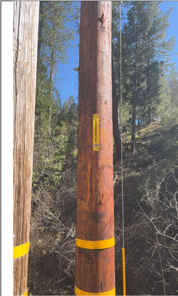
Photo 1: Photo of pole ID 122368402 located approximately 27 feet south of the subject tree.
