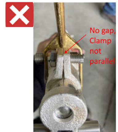
Figure 19 Improper End Fitting Installation
