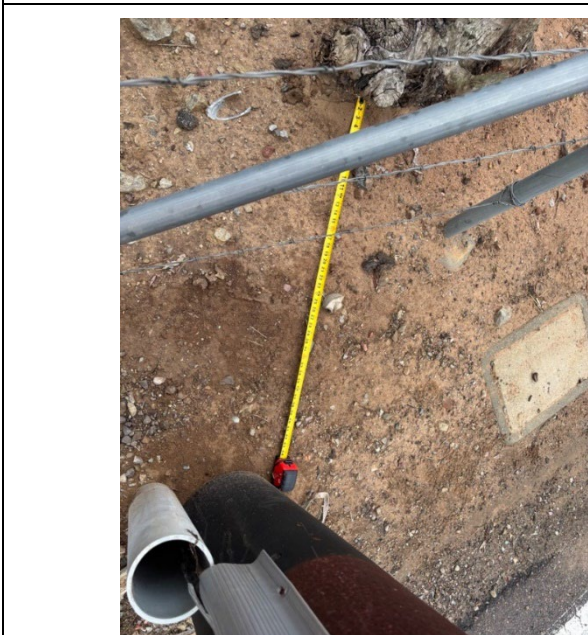
Photo 3: Measurement shows one of the two eucalyptus stumps located approximately four feet from the base of the pole.
