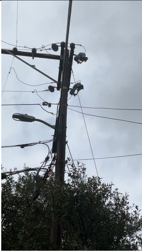
IA1Img3: Solid Blade Disconnects and lack of reclosers, sectionalizers, or voltage regulators.
