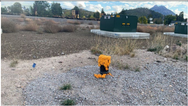
IA1mg1: No distribution pole at this location
