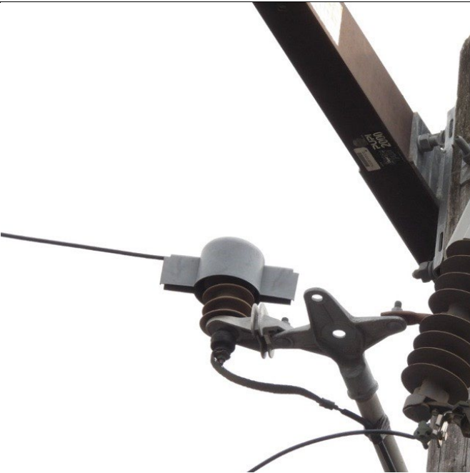
Photo 5: Close-up image of non-exempt surge arrester on the pole.
