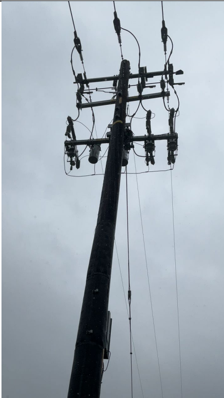
IA1mg1: Southeast view of pole 121774370
